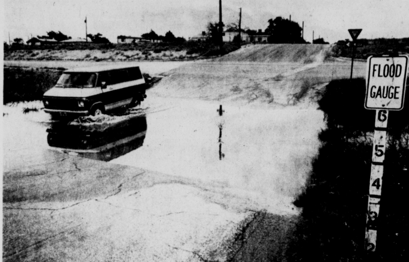
Some streets in Midland are more subject to water damage than others. Here, Edwards Street — which passes through Scharbauer Draw — is filled with water from recent rains. (Staff Photo)
