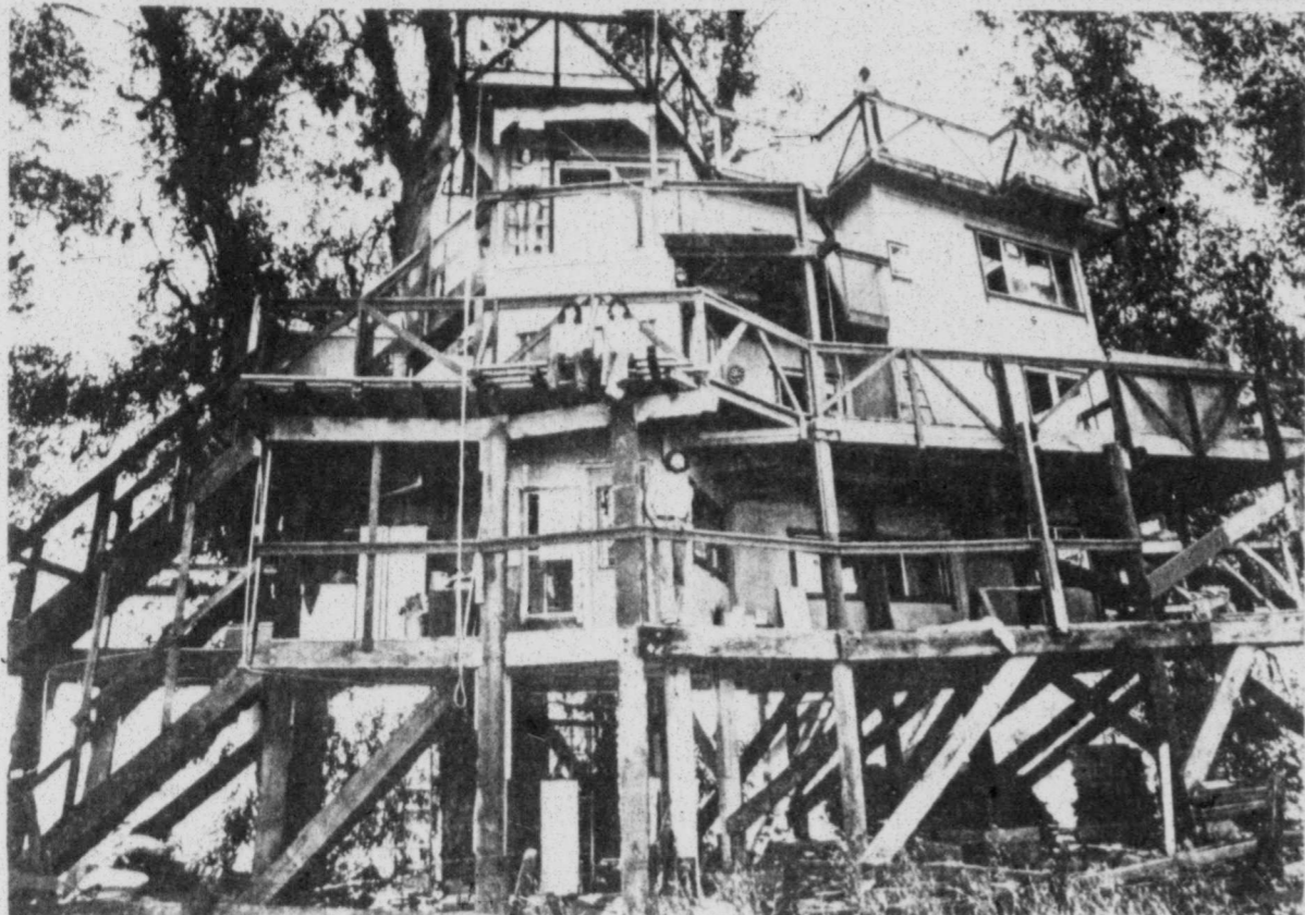
Professor Glen Gaviglio's 4-story, 11-room tree house is supported by five eucalyptus trees and 19 pilings. It has four bedrooms, two bathrooms, a hot tub and an all-electric kitchen. (Los Angeles Times Photo by Fitzgerald Whitney)
