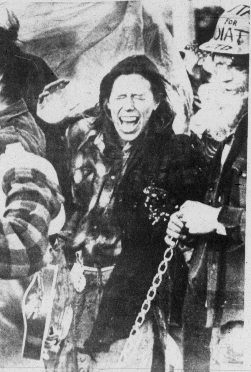
A demonstrator from Maine reacts as she is hit in the face with Mace sprayed by police through the front fence of the Seabrook nuclear power plant construction site Monday evening.
