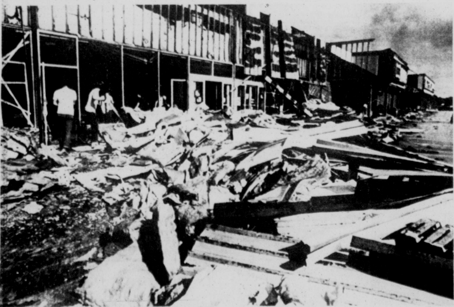
Workers pull debris from a supermarket in Pensacola, Fla., that was hit by the high winds of Hurricane Frederic Thursday. (AP Laserphoto)
