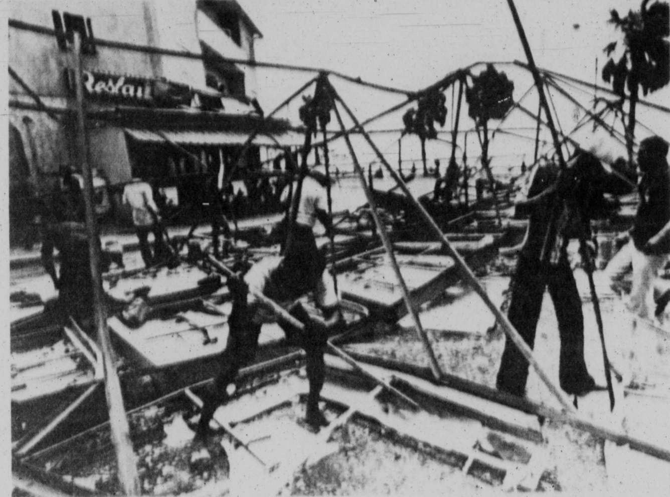
Residents of Santo Domingo try to raise heavy steel beams, blown down by the strong winds of Hurricane David. The entire city suffered heavy wind damage. Many of the people were in the streets Sunday helping with the clean up, and digging bodies out of the rubble.
