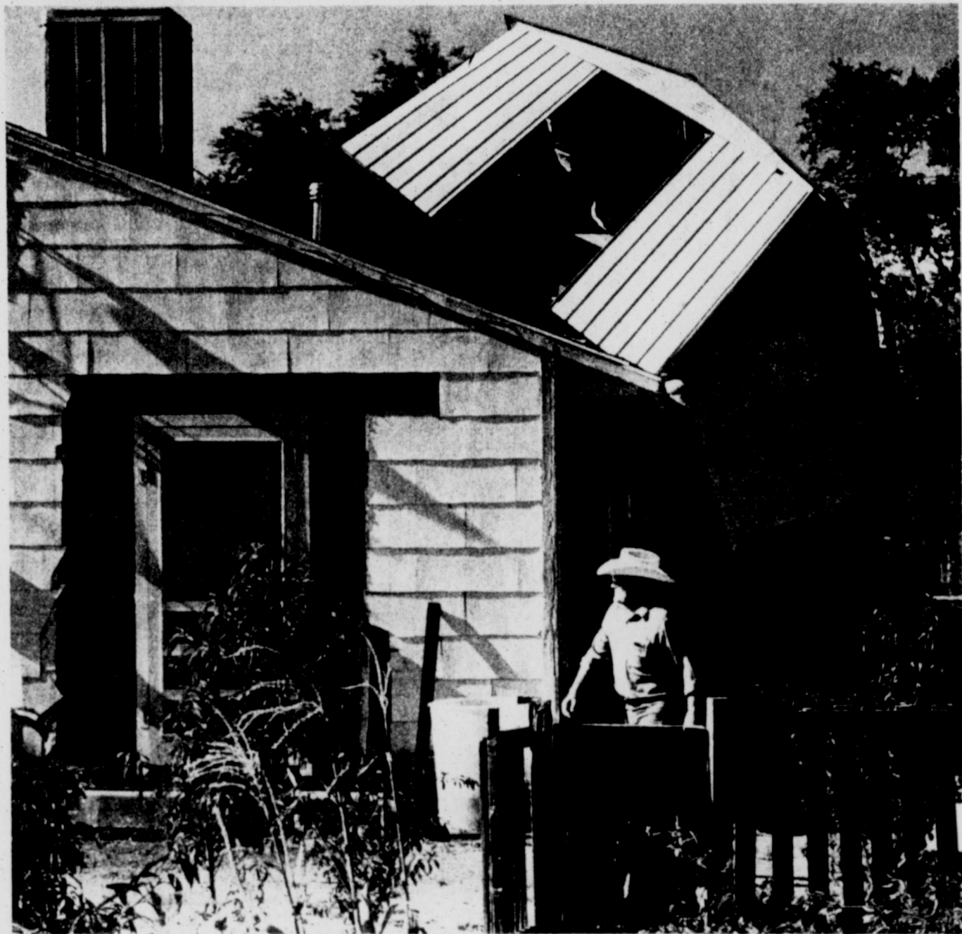
High winds Thursday added a temporary second story to a building at 701 S. Pecos St. occupied by Busy Bee Plumbing and Supply and the Midland Gem and Mineral Society. A metal storage shed
