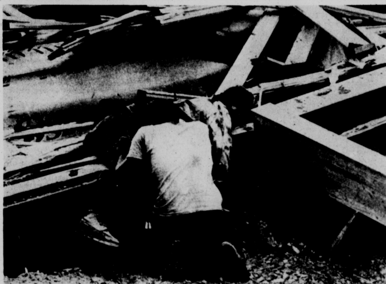
A construction worker weeps beside the body of his friend following Monday's collapse of a sports stadium under construction in Rosemont, Ill. In-
