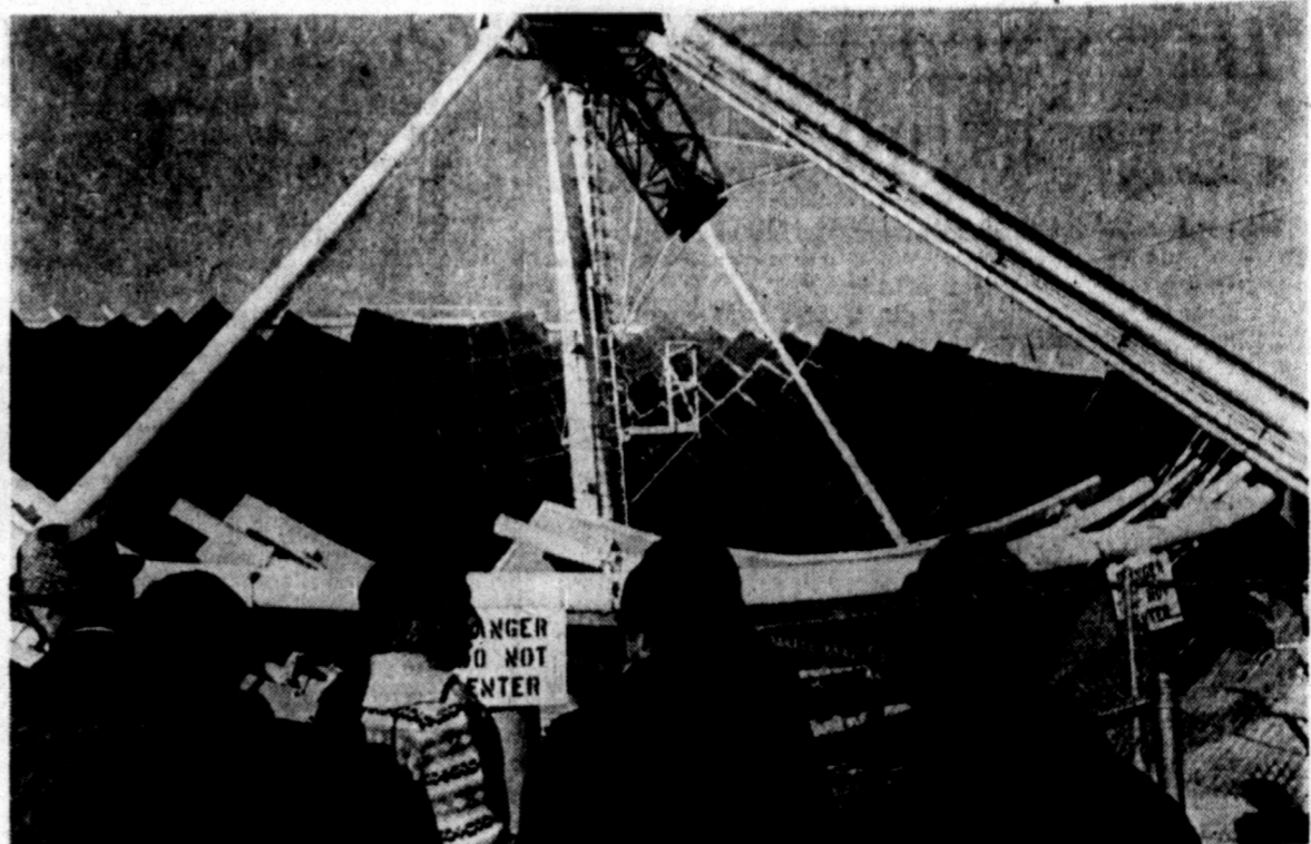
SOLAR STEAM MACHINE — The Crosbyton Solar Power Project, designed to help Crosbyton residents reduce their energy costs through solar power, took another step toward completion this week when the first blast of steam was produced at the site. The sunlight collected in this 65-foot diameter mirrored dish heats water to produce steam which scientists say can be harnessed to produce electricity. (Staff Photo by Bill Janscha)
