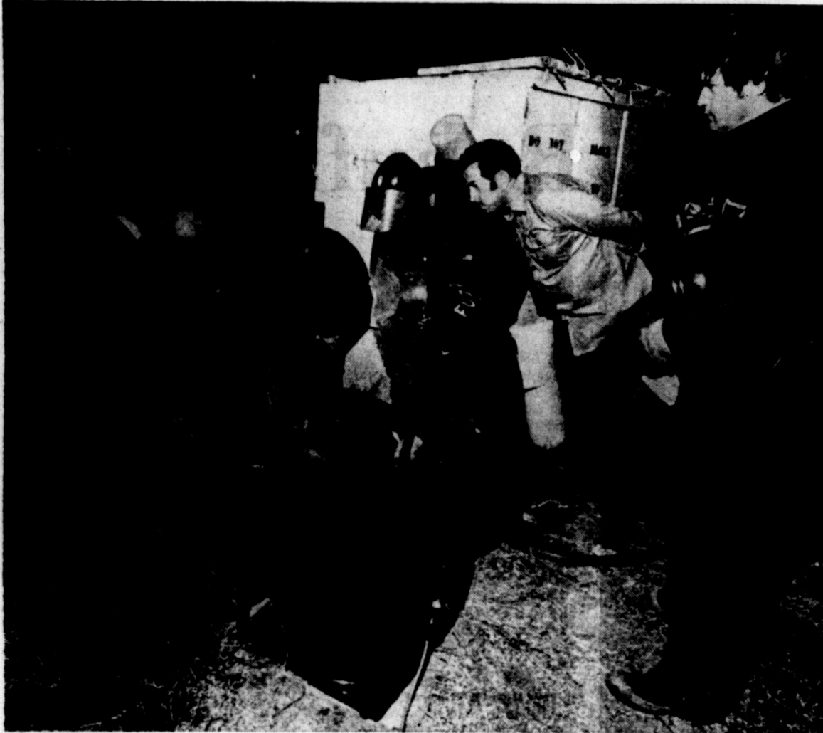
FIRE IN THE HOLE —A fire in a manhole near the Ranching Heritage Center of the Texas Tech Museum attracts quite a crowd of firemen just before dawn today. The blaze, apparently
