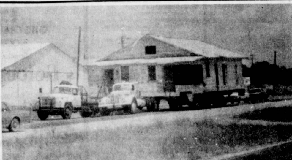
HOUSE TROUBLES- Vernon Honea and company of Cisco were moving the house shown from Eastland along Hwy. 80 when they ran into some trouble just outside of Cisco near the old Terra Firma Tile plant. The building apparently lost its support underneath the right side and tilted over until it was resting on the highway shoulder. The professional movers they are, Honea and company returned to Cisco for more winch trucks and had the house lifted and were preparing to move it again when the above photo was taken. (staff photo)
