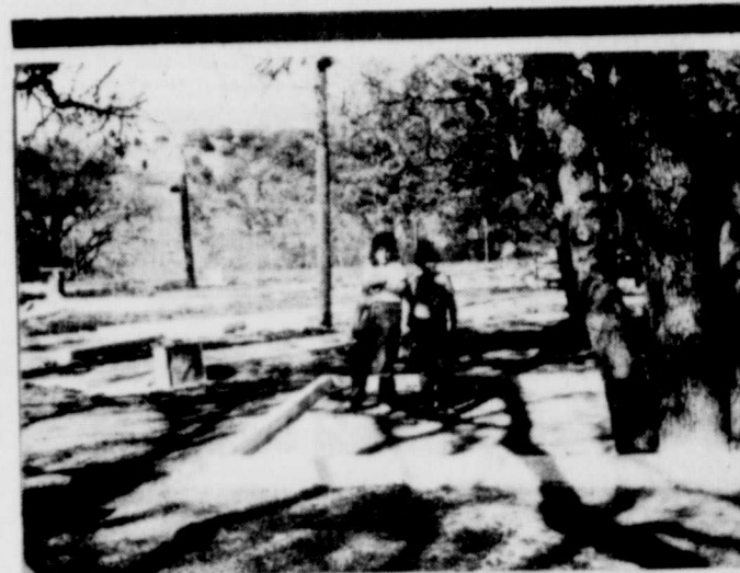
Danielle and Cullen Rabel lend a helping hand to renovate the old miniature golf course at Lake Cisco Park. The Kiwanis Club is sponsoring the renovation and reopening of the course.
