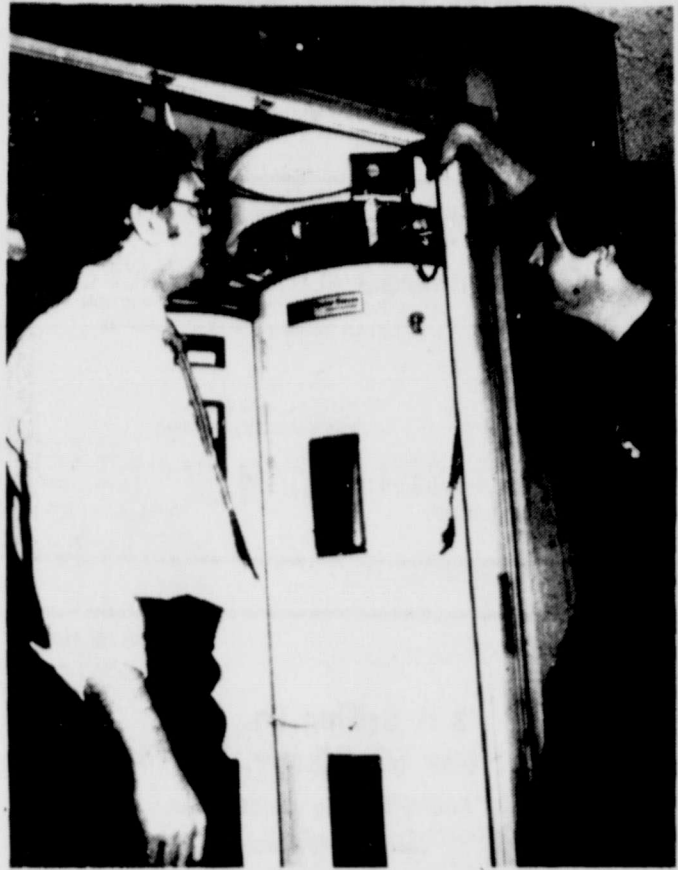
INSPECTING the 80-gallon water tank that is part of the new Reynolds Aluminum Solar water heating system at the Hogan home are Gail Hogan, left, S&M Supply Co. official, and Roy L. Griessmyer of Dallas, district manager for the Reynolds energy products group. The system was installed at the Hogan home during the past week. (Staff Photo)
