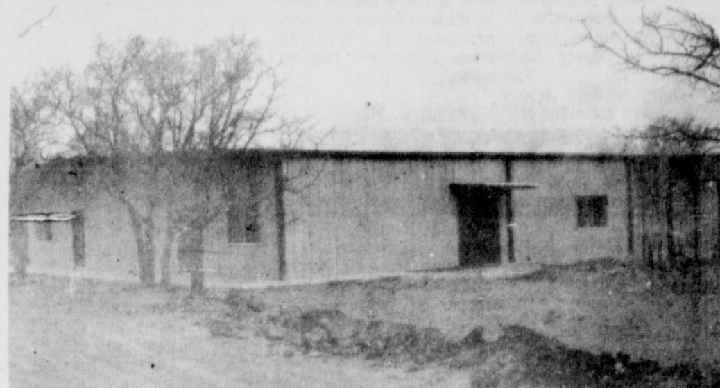
The new all-purpose building at the Lake Cisco Christian Camp is shown above. It was erected at the camp at a cost of about $100,000. It will seat up to 330 people for meetings and houses a cafeteria, kitchen, infirmary, rest rooms and other facilities. (Staff Photo)
