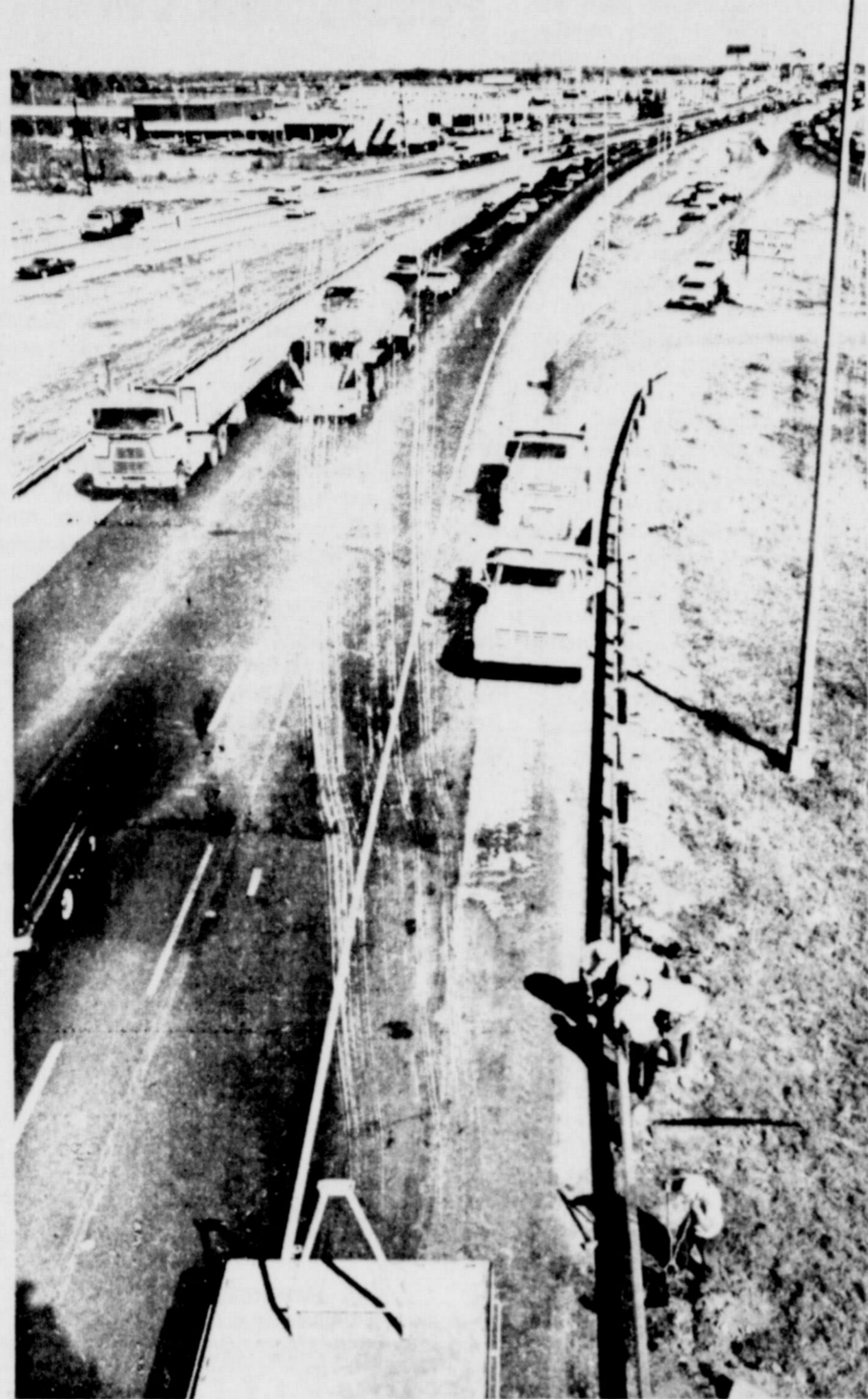
These highway workers stake their lives on the skills of 50,000 drivers during one day of maintenance work on freeway guardrails.
