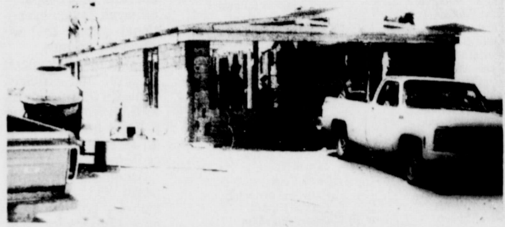
Local people help build parsonage in Mexico
