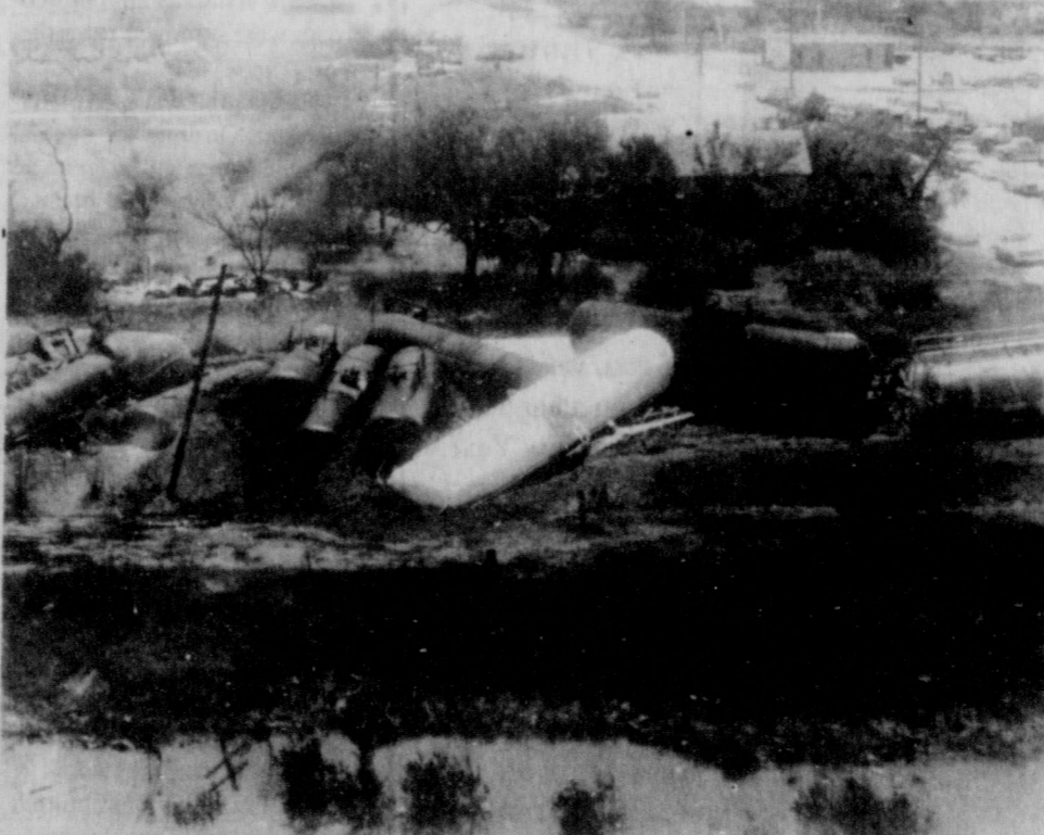
Smoke finally clears after the May 24, 1985 train derailment near North Seaman St. in Eastland, revealing ruptured tank cars. This big Eastland County story was carried on national news networks.
