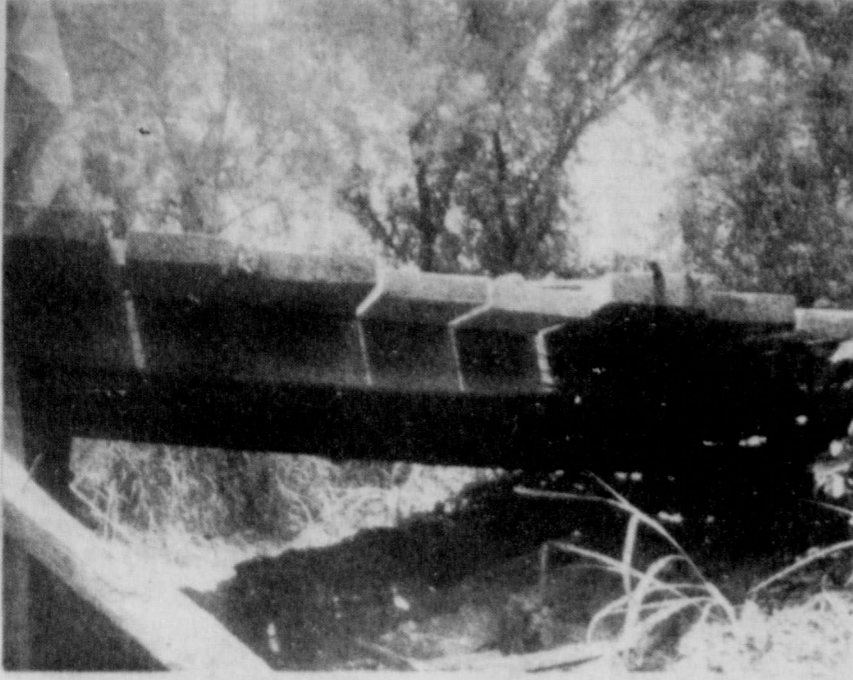
Time for some work! This old bridge was getting shaky.
