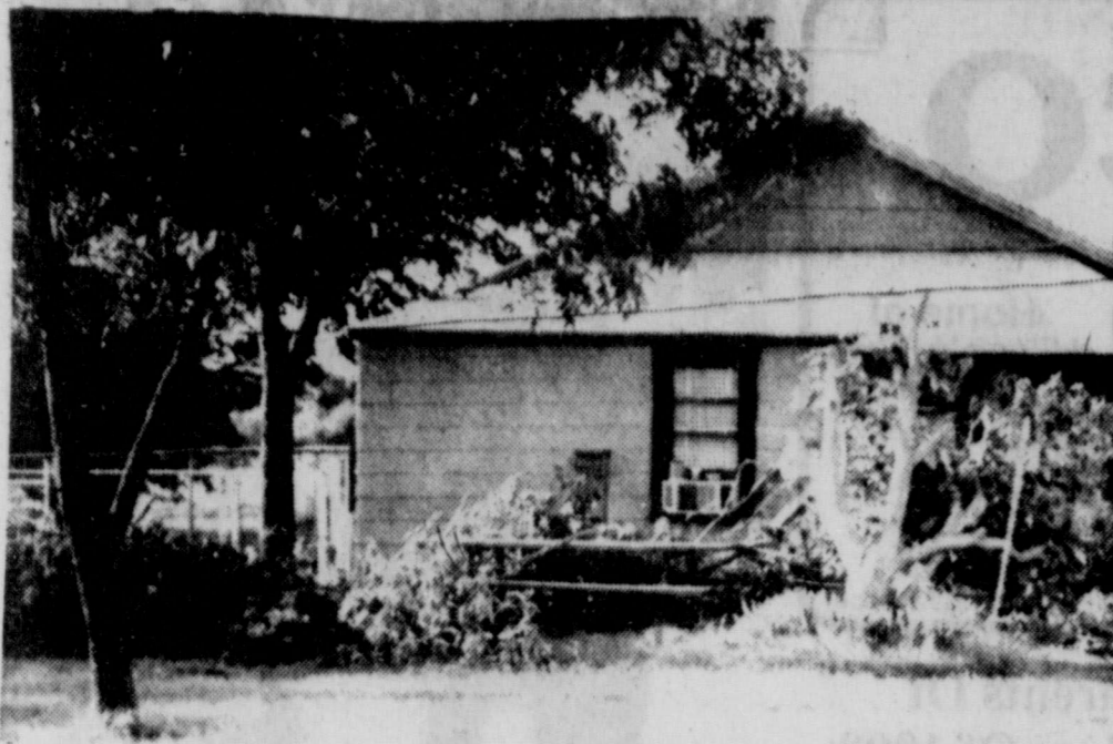
Fallen tree in back yard in home on West 17th Street.
