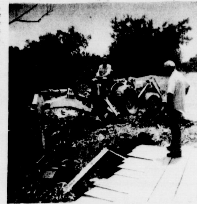
Larry Green operates the equipment while Comm. Bacon looks off the new bridge.
