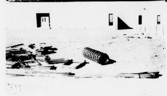
CONSTRUCTION-- Work has begun at the Cisco Elementary to build a new gym on the west side of the school. Iron rods and wire are shown in the above photo, ready to be placed down so the cement can be poured for the floor. Brownwood Construction has the contract for the new building. It is estimated that the gym will be completed by September, 1988. (Staff Photo)
