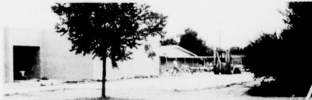
The old Cisco Intermediate School is gone now and the new Cisco Elementary School is almost finished. A circular drive will be in the above location by September.
