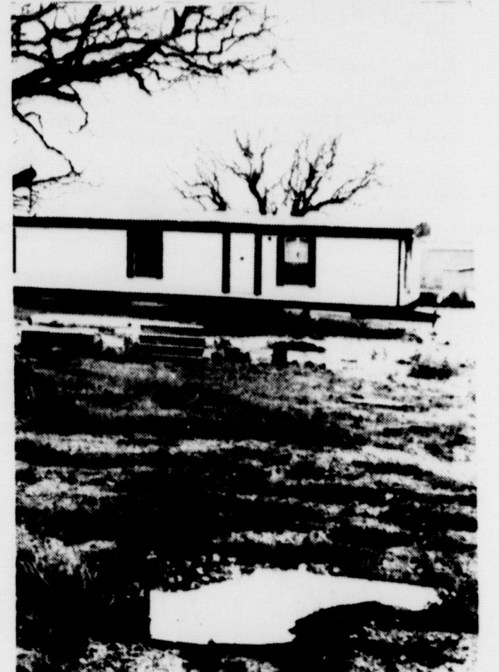
STORM DAMAGE - A trailer home suffered extensive damage when it was rolled by high winds Wednesday night. The trailer landed atop a generator and against a tree and was considered a total loss at the Carroll Electric Co. on Hwy. 69.
