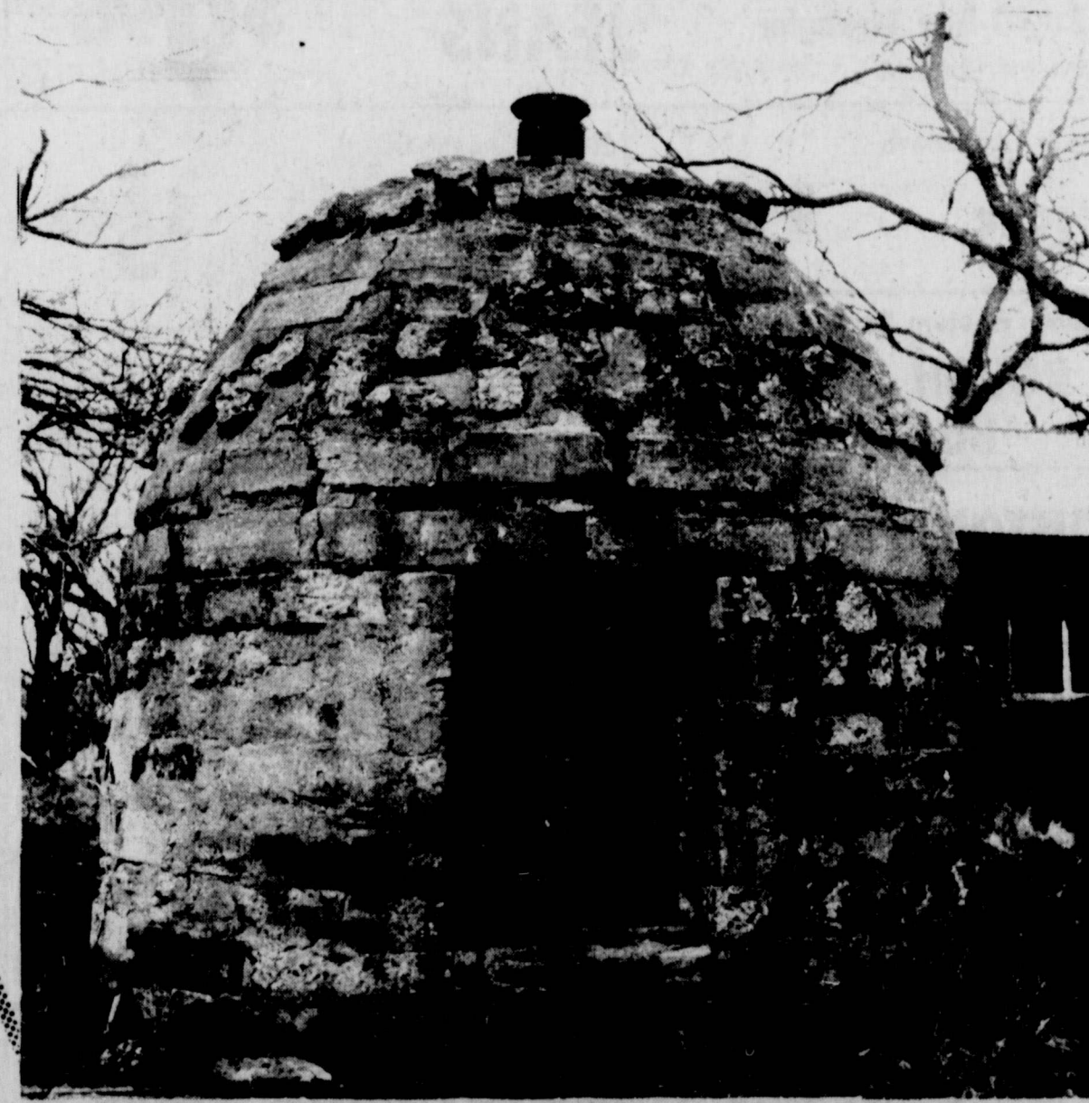
WELL DONE?—How do you like your wood—Mesquite, that is—medium, rare? Or, well done? This wood drying kiln built by a man named Loving about 1930, with help from John Chalker, still
