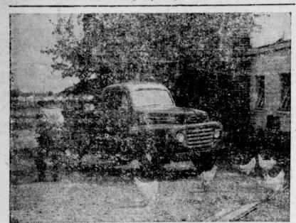
SERIES F-3 1950 model Ford truck with stake body. Maximum gross vehicle weight rating is 6,800 pounds. An eight-foot express body also is provided. One of 175 new 1950 mode. Ford trucks.
