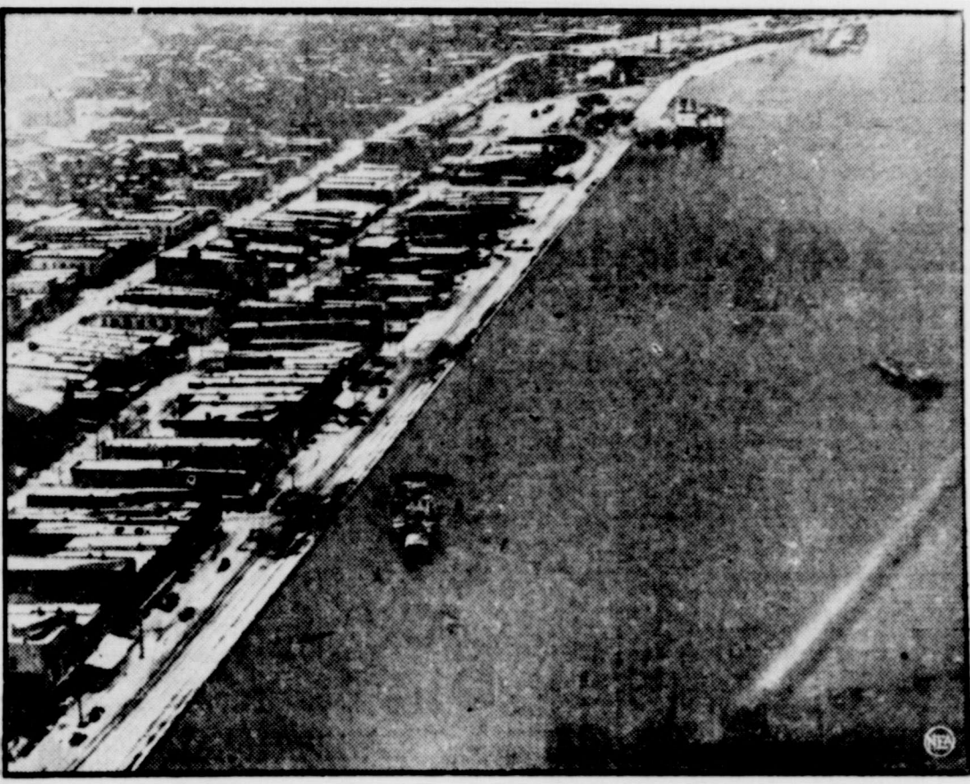
The thin line of levee on which hung the hopes of Cairo, Ill., today as the Ohio river water lapped at the levee. The Ohio air waters taken the very top of the 60-foot wall. The boats shown along the levee stand higher than the roof-tops of the buildings along the street. Facing this terror, women and children were evacuated, men remained to strengthen the levee as pressure of the river water oiled up through holes in the pavements, and fissures and cracks kept appearing in the levee itself.
