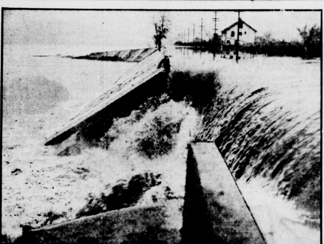
Through this huge gap ripped in Bechnout levee, Cincinnati by the Ohio river's pounding flood waters a roaring torrent poured down on lowlands, converting them into a shallow sea and inundating Lunken airport. Even the higher land seen in the background the water rose to a threatening level, in the third greatest deluge in Cincinnati's history.
