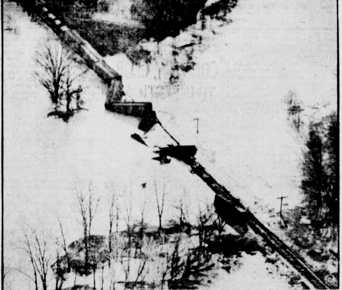
Derailed when the surging waters of the Cumberland river undermined the Louisville & Nashville railroad tracks near Palmyra, Tenn., 15 cars of this freight train were spilled into the torrent causing heavy damage. This picture, taken from the air, shows the remainder of the train still on the rails and all the surrounding area submerged. Service on the L & N main line from Bowling Green, Ky., to Memphis, Tenn., was delayed by the disaster.
