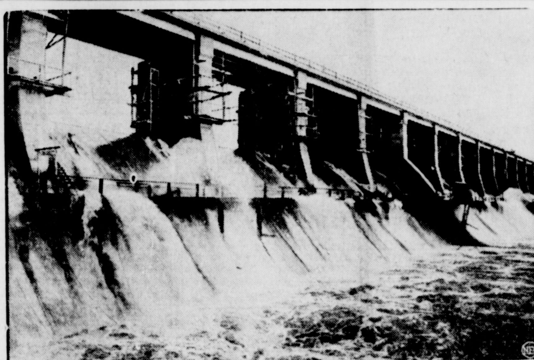
Given the initial test of its flood control value by the torrents that raged over North Carolina, Tennessee, and Alabama, Wheeler dam is shown here as water poured over its spillways for the first time. The spillway section of the giant TVA barrier on the Tennessee river is 43 feet high. By raising the gates, 15 feet can be added. The dam will be completed by the end of this year.
