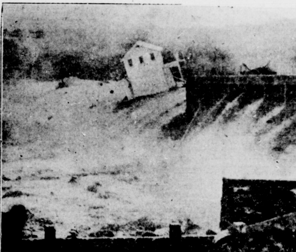
Flood waters sweep house over dam at Lake Austin.
