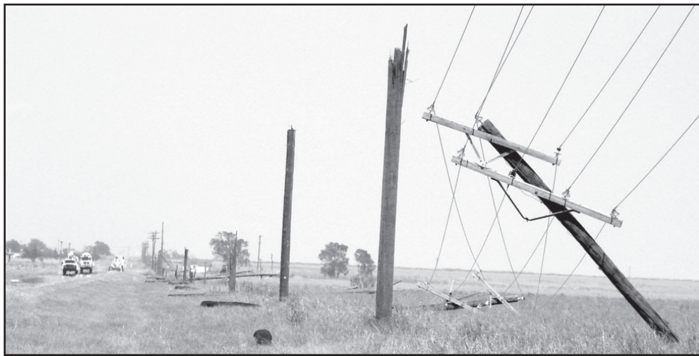
BCEC's recent storm damage included more than 400 utility poles. Pictured above, the power lines hold up the pole, while below linemen arrive at a damage area.
