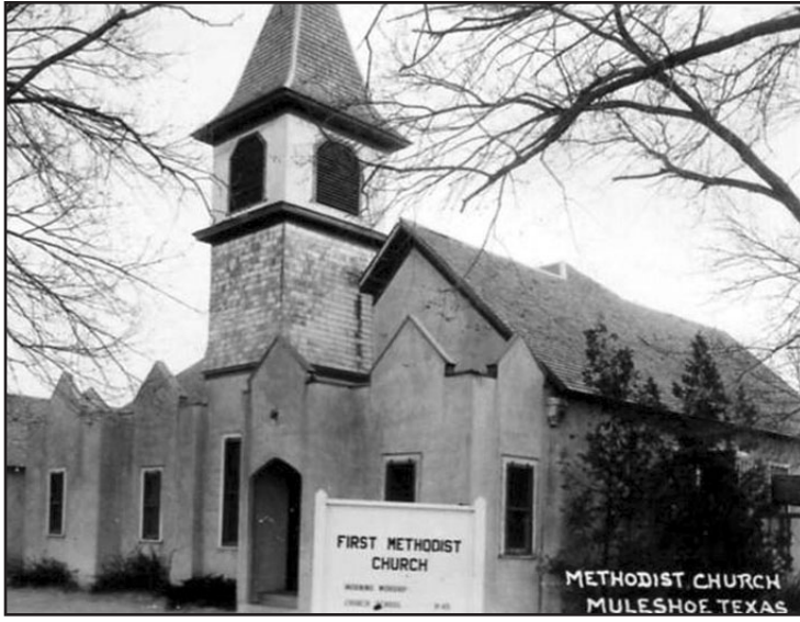
The "Old Hurley" Church after the move into town, with additions and a stucco exterior.
