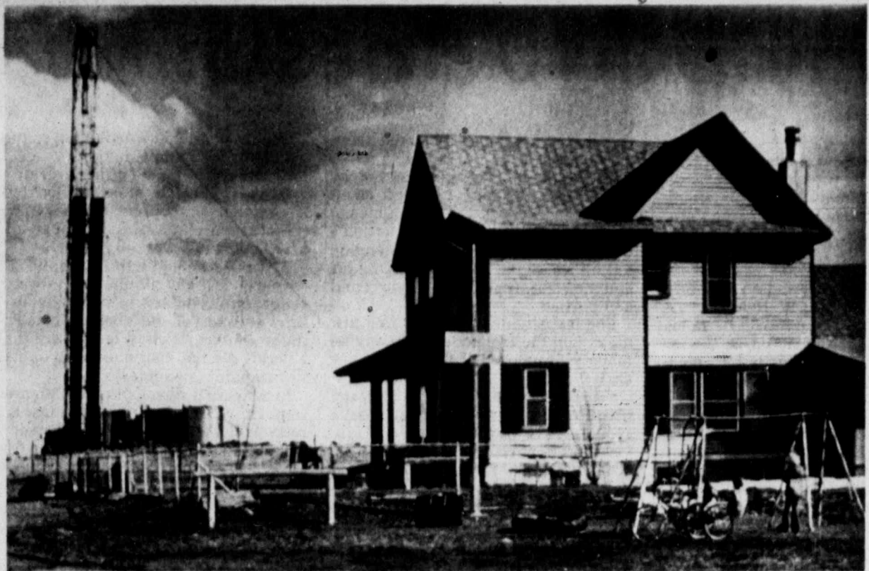
Development of energy resources is changing the wide-open spaces of Wyoming and creating some problems too. A Denver oil company purchased mineral rights and
