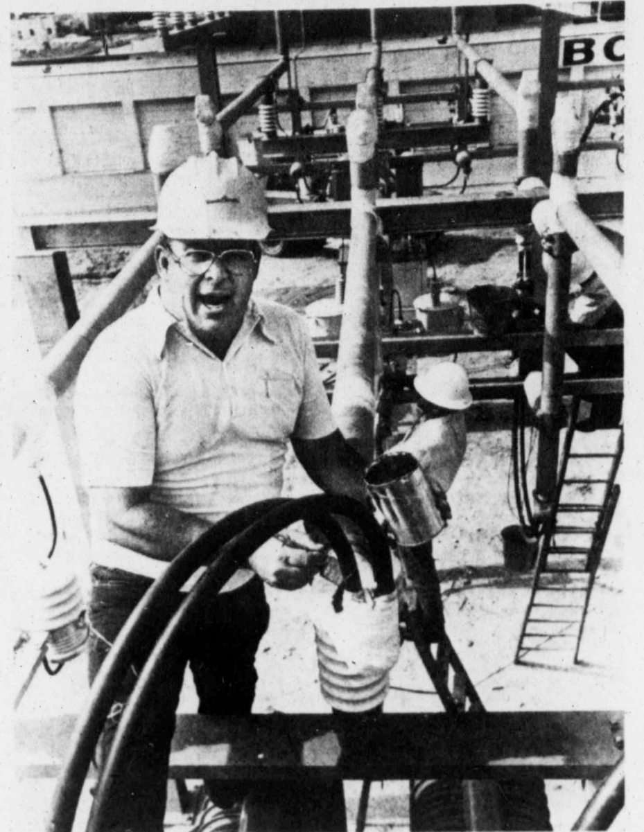
"We shouldn't have the problems here we've had at other Midland substations," explains TESCO electrician L.A. King. King and fellow worker Troy Jones, in background, are wrapping all exposed contact points near the transformer being constructed at Washington and Colorado streets with fiberglass to avoid shorts caused by animals and vandalism. (Staff Photo by Bruce Partain)
