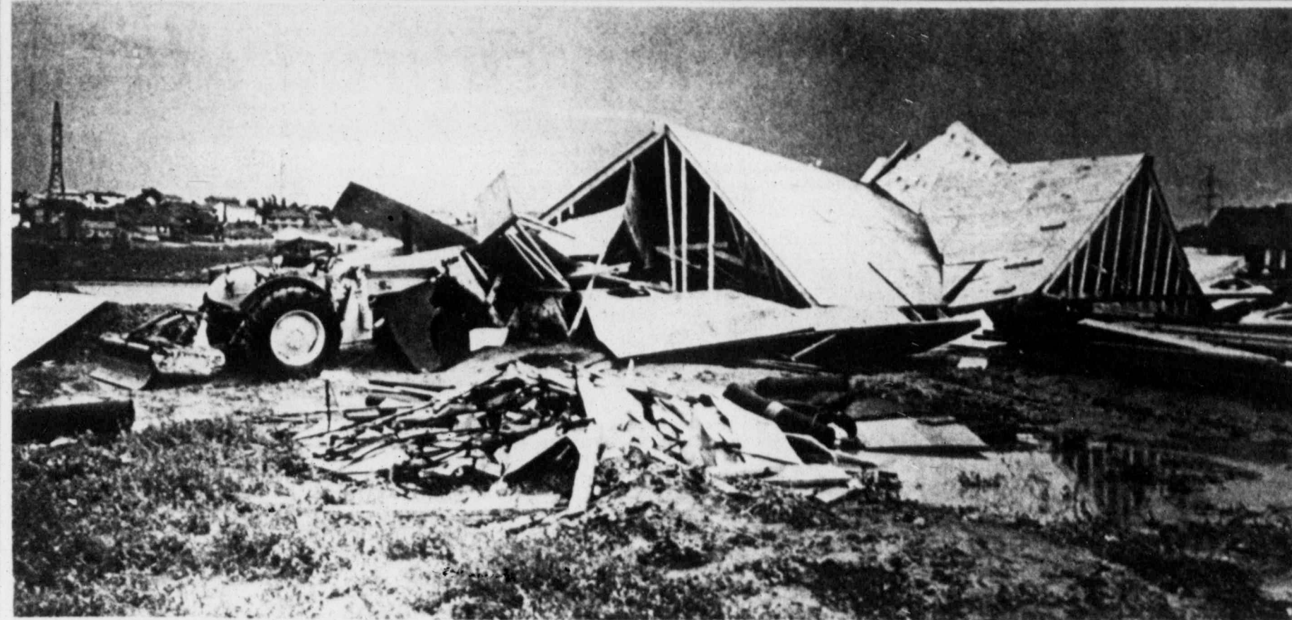
A house under construction in southwest Omaha, Neb., was leveled by strong winds Tuesday as turbulent weather struck 23 counties of eastern Nebraska. Two men in the small community of Oakdale were killed when winds struck a metal shed in which they were working. (AP Laserphoto)
