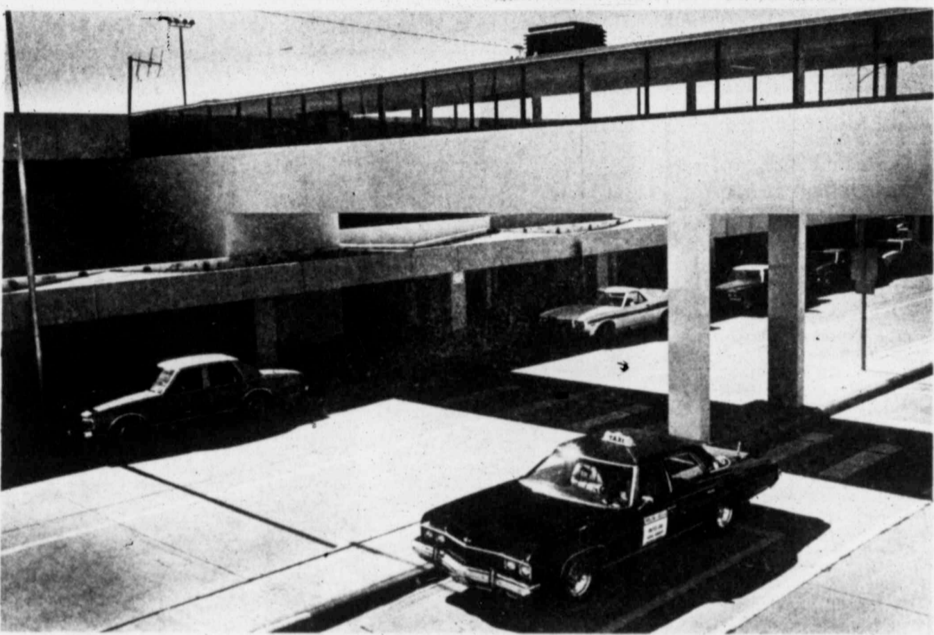
An enclosed walkway from the second floor of the parking lot to the completed terminal facility at Midland Regional Airport keeps passengers out of
