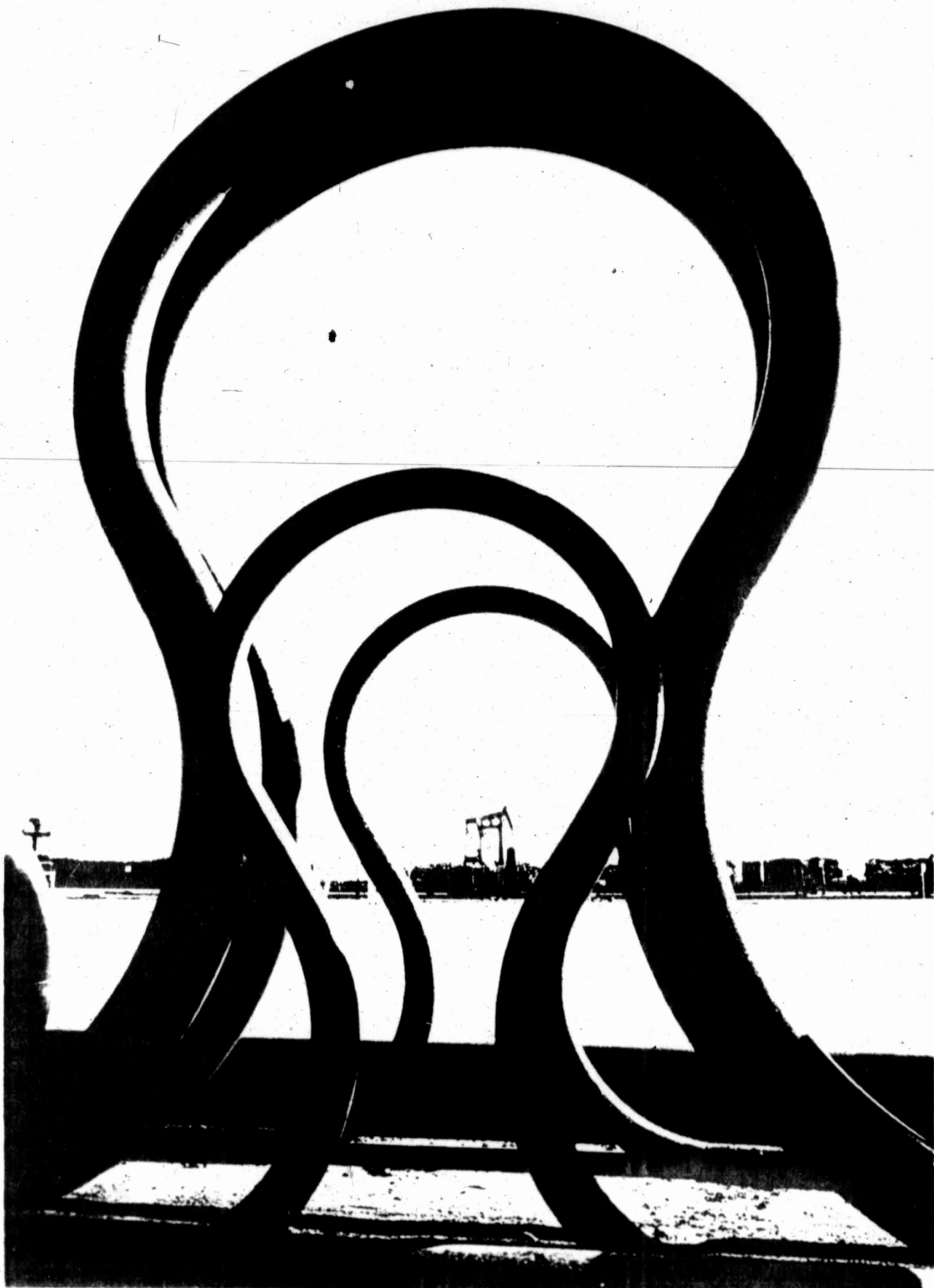
Although they ignore the axiom that the shortest distance between two points is a straight line, these pipelines at Aminoil USA's Huntington Beach, Calif., production facilities, were designed, nevertheless, with function in mind. The graceful bulges give the pipelines the flexibility to contract and expand as temperatures vary without causing damage.
