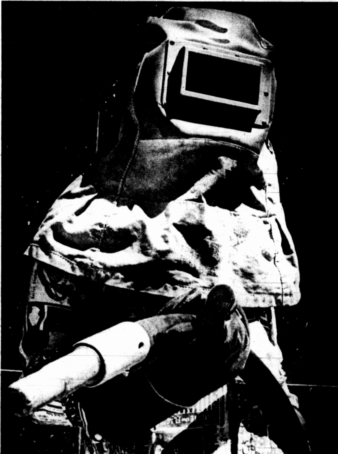
A strangely garbed figure, looking not unlike a space traveler and seen prowling Big Spring Street this week, turned out to be Charlie Alsheimer, who was sandblasting sidewalks surrounding First National Bank. (Staff Photo by Bruce Partain)
