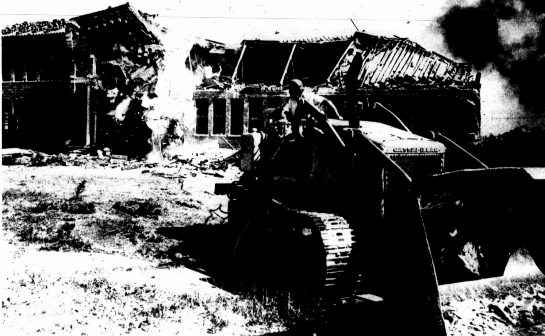
The walls of North Elementary School come tumbling down Tuesday as Bennie Doggett, Lubbock demolition specialist, fulfills every
