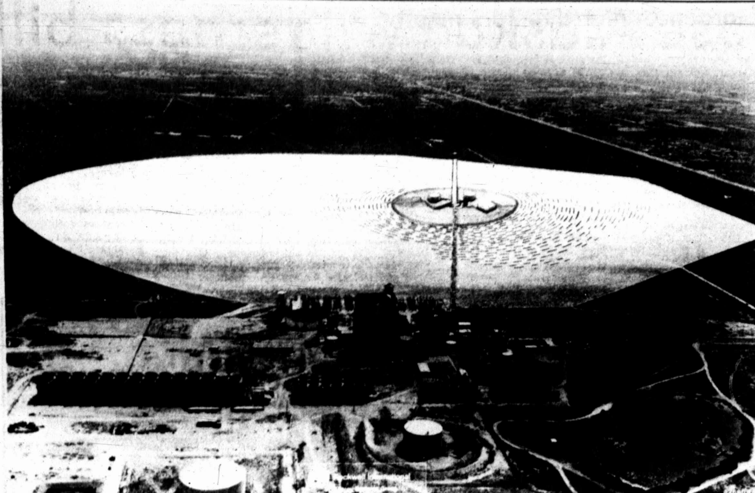
Texas Electric's Permian Basin power plant near Monahans is shown with a proposed solar energy system superimposed where it might be located. TESCO, along with Rockwell International, is applying for federal approval to study the concept of converting an existing gas-fired unit to use solar energy.
