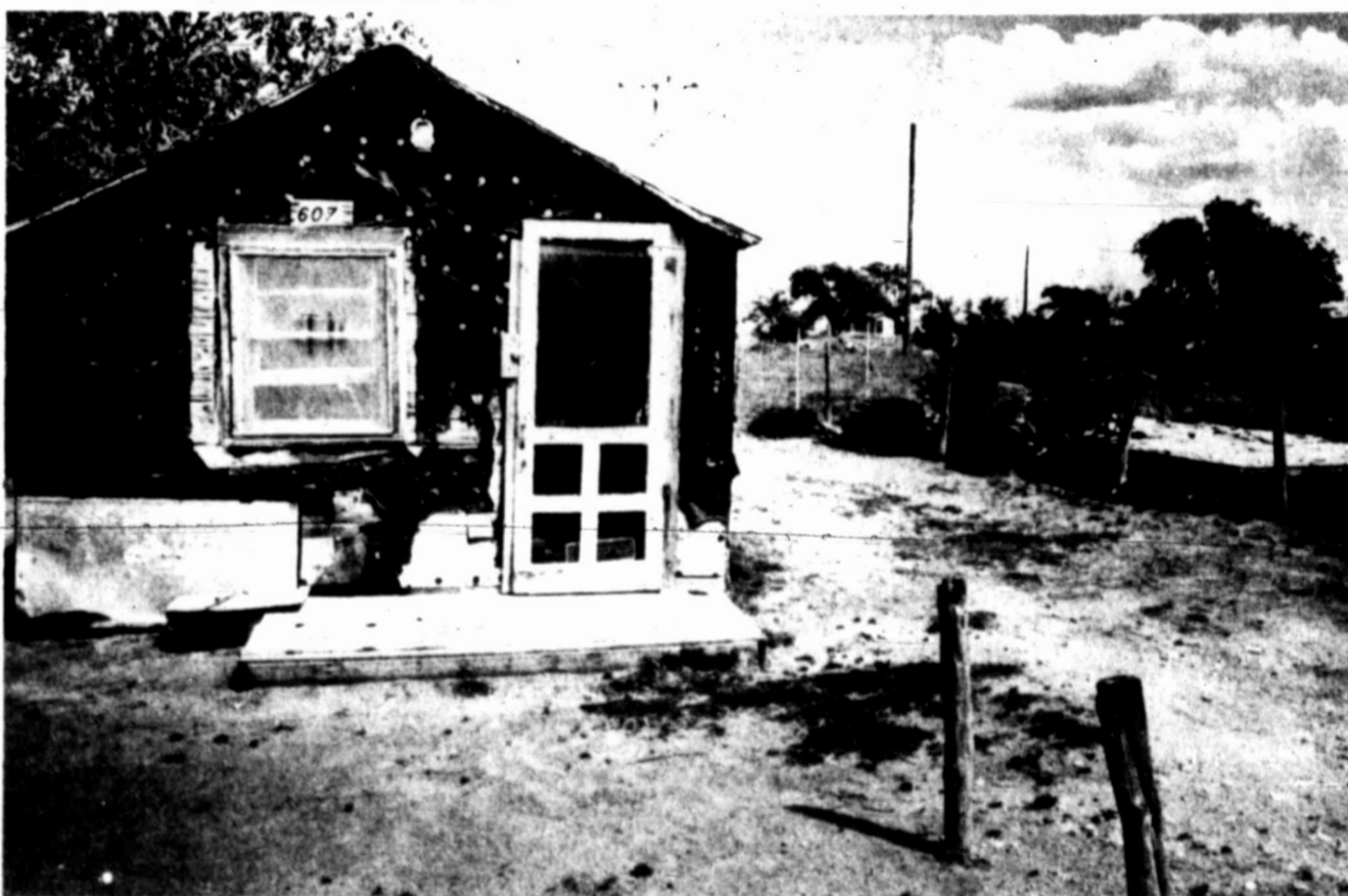
Sitting on its south Midland plot of land since 1948 is this two-room house owned by Lois Gray. Like many of Midland's senior citizens, Mrs. Gray lives on a fixed income and finds it difficult to keep up repairs on her two-room house. (Staff Photo by Mike Kardos)
