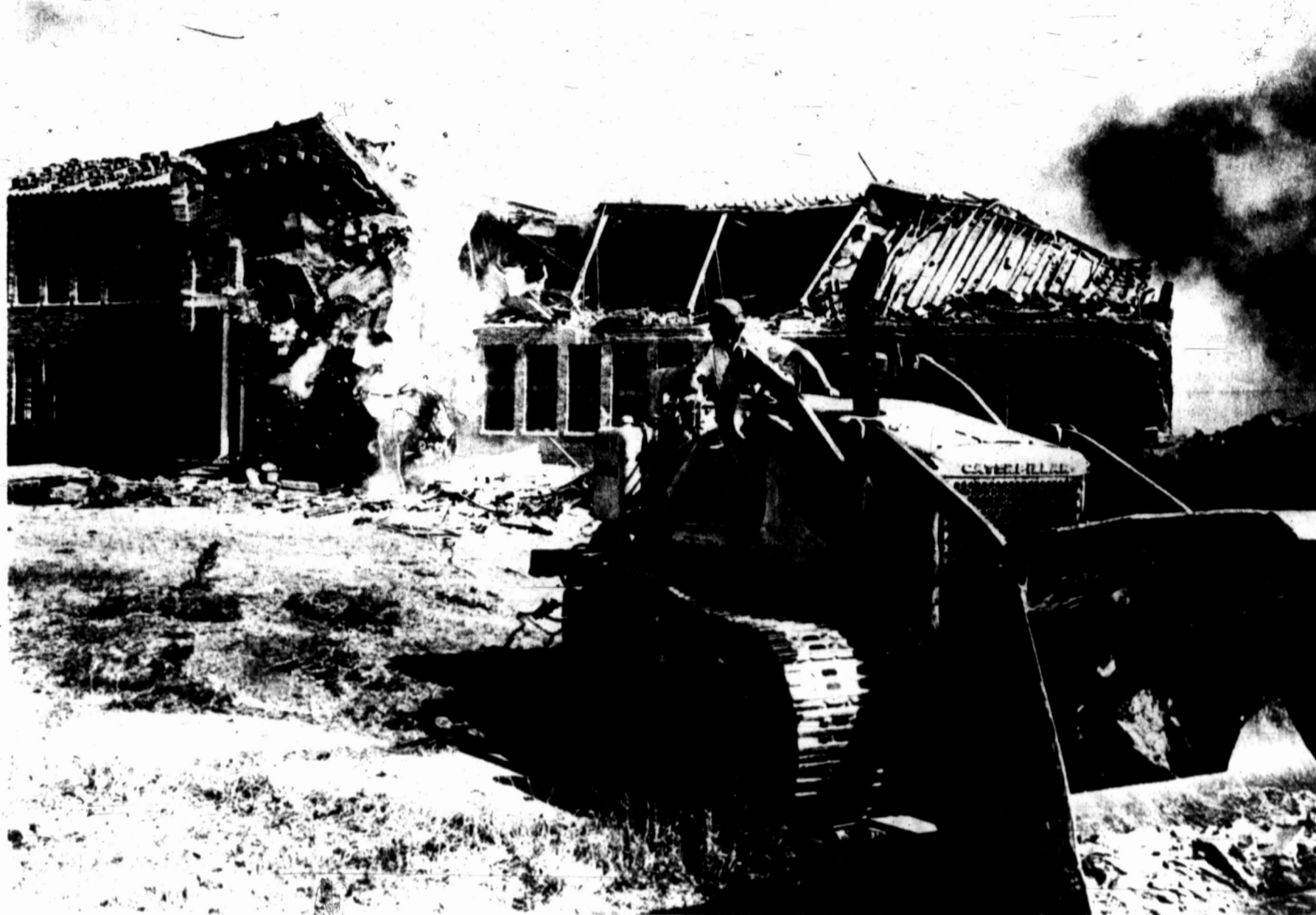
The walls of North Elementary School come tumbling down Tuesday as Bennie Doggett, Lubbock demolition specialist, fulfills every schoolboy's fantasy of how school should really end. A demolition crew has contracted to have the 42-year-old building cleared away by the end of May.
