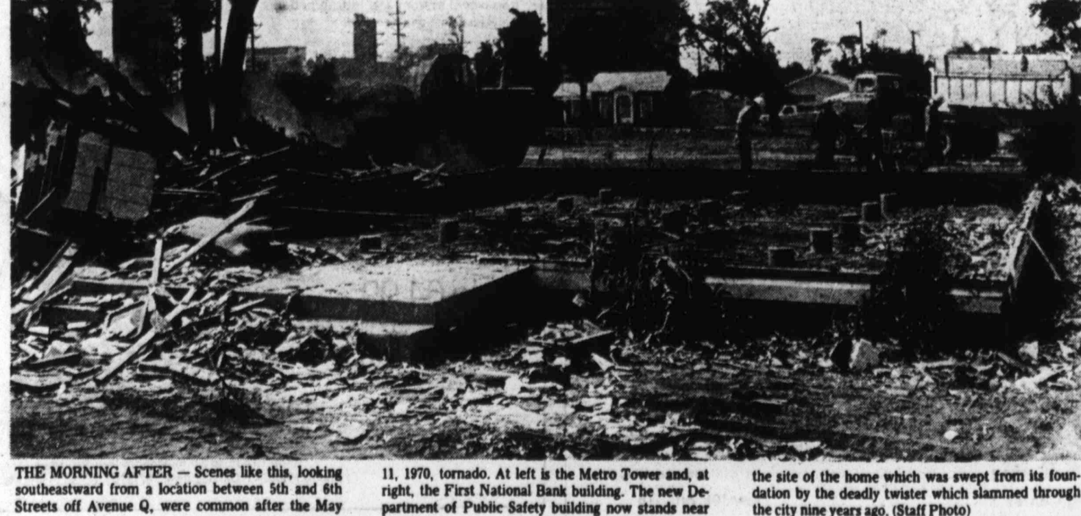
THE MORNING AFTER — Scenes like this, looking southeastward from a location between 5th and 6th Streets off Avenue Q, were common after the May 11, 1970, tornado. At left is the Metro Tower and, at right, the First National Bank building. The new Department of Public Safety building now stands near the site of the home which was swept from its foundation by the deadly twister which slammed through the city nine years ago. (Staff Photo)
