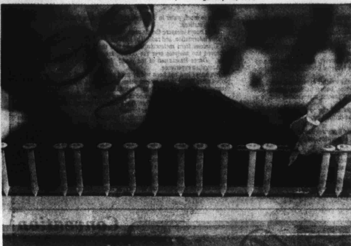
NOT GOLF TEES — What looks like golf tees at first glance are actually pop-up temperature gauges undergoing quality control inspection at a 3M Company in Fresno, Calif. The gauges, pointed at one end, are inserted into turkey, chicken
