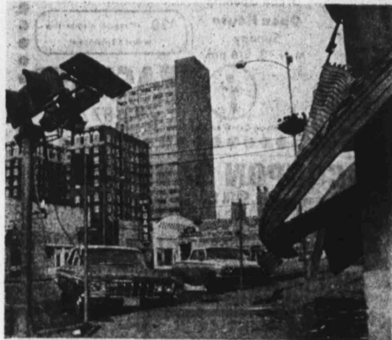
DOWNTOWN DAMAGED — The Lubbock tornado left twisted signs and mangled buildings in its deadly wake. This photo, looking north from Main Street and Avenue J, shows the damage done to the Lindsey Theater marquee and the Great Plains Life Building, which was twisted almost to the point of being unsalvageable. (Staff photo).
