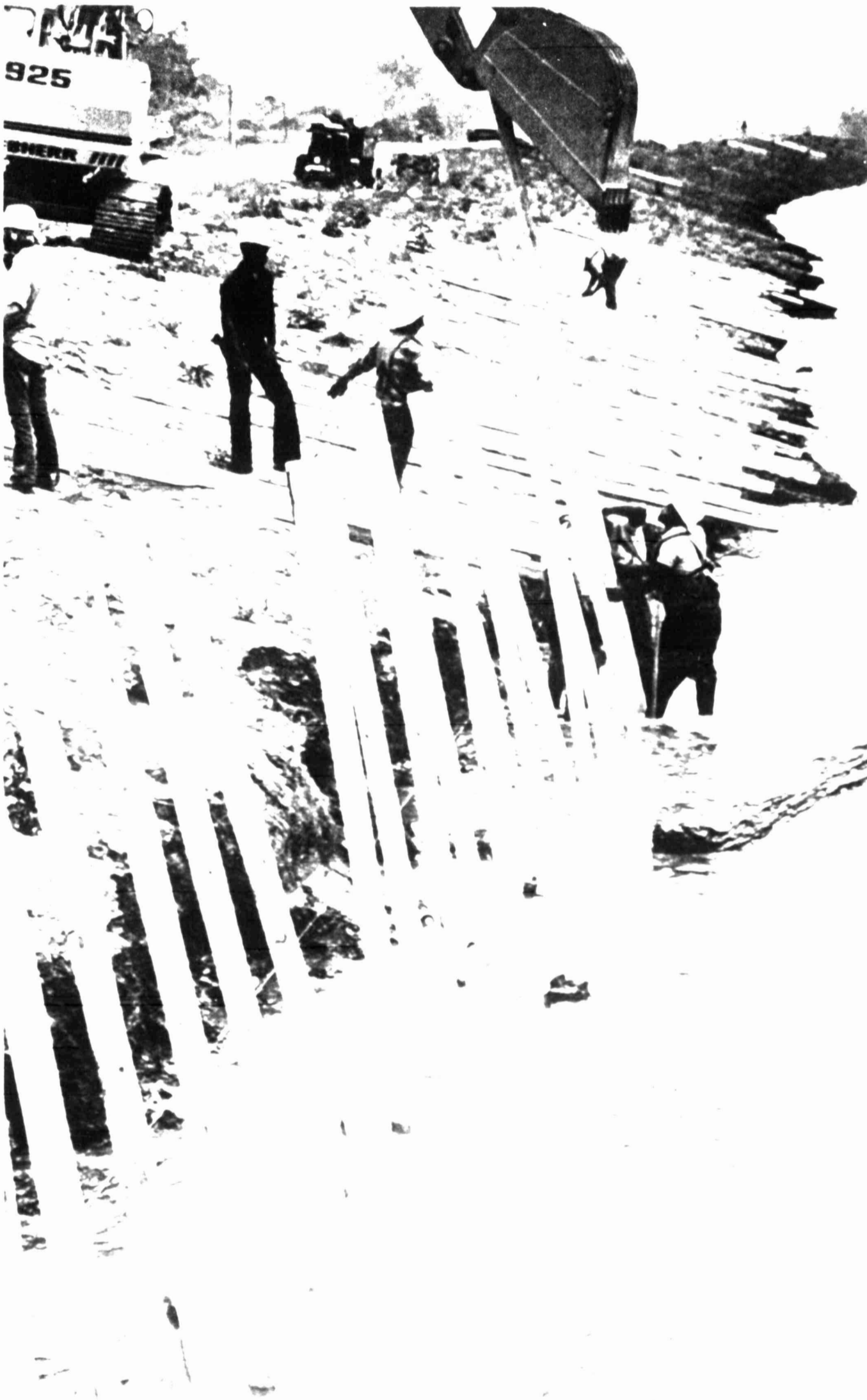
Workers spent the weekend erecting a board fence along a 1,900-foot section of the Mississippi River levee in Baton Rouge, La. The fence, intended to stop erosion of the levee by high water, will
