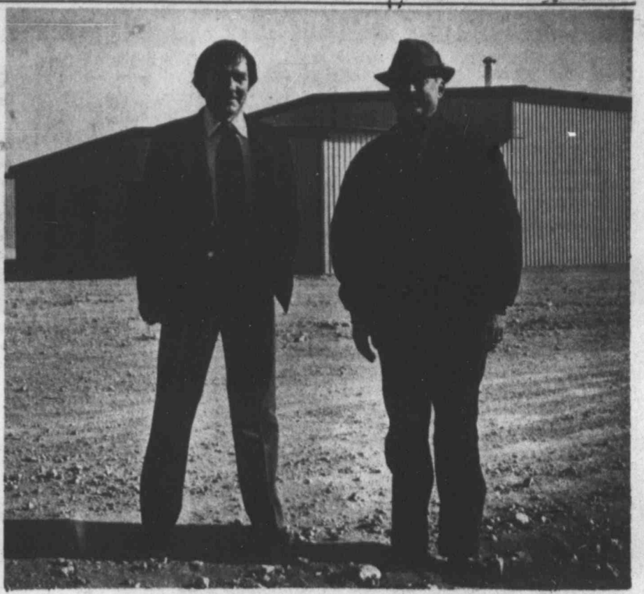
Tom King and Bill Chancellor, on the site of their planned industrial area located on Francis Street west of Cottonflat Road, are proud of the new warehouse ready for sale. It has a paneled 20x50 office with central air, is insulated and has skylights, overhead heaters and is served with gas and electricity. County zoning with city convenience. Call Tom King, 682-6000, or Bill Chancellor, 683-2040.
