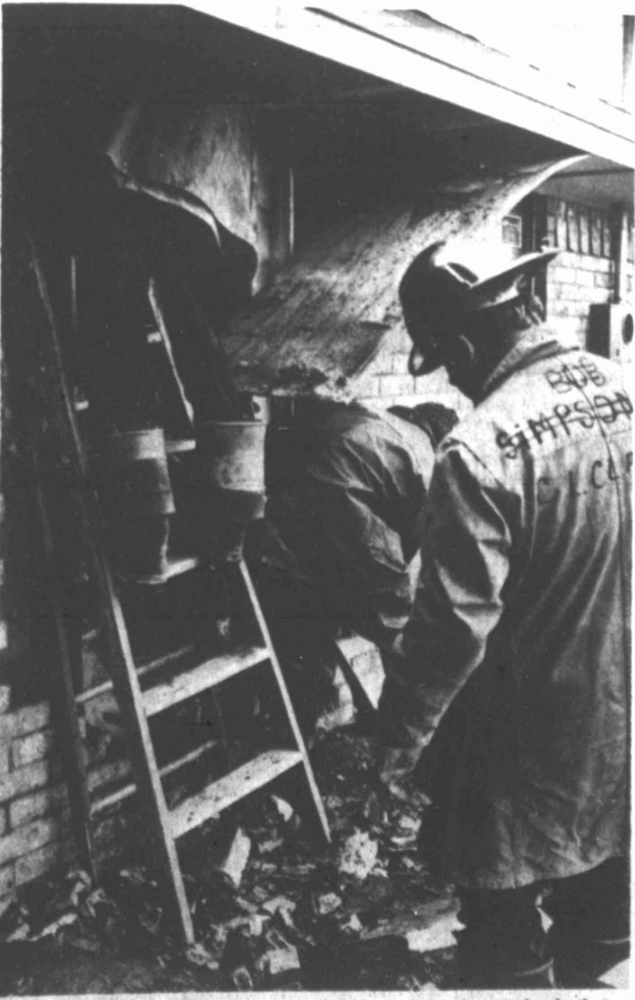
Firefighters sort through the rubble and begin to check the interior of the roof of a house which was under construction when it caught fire Friday. Officials said workers at the house, in the 2600 block of Mark Lane, had built a fire in the fireplace, when heat apparently ignited materials in the house and roof. (Staff Photo by Mike Kardos)
