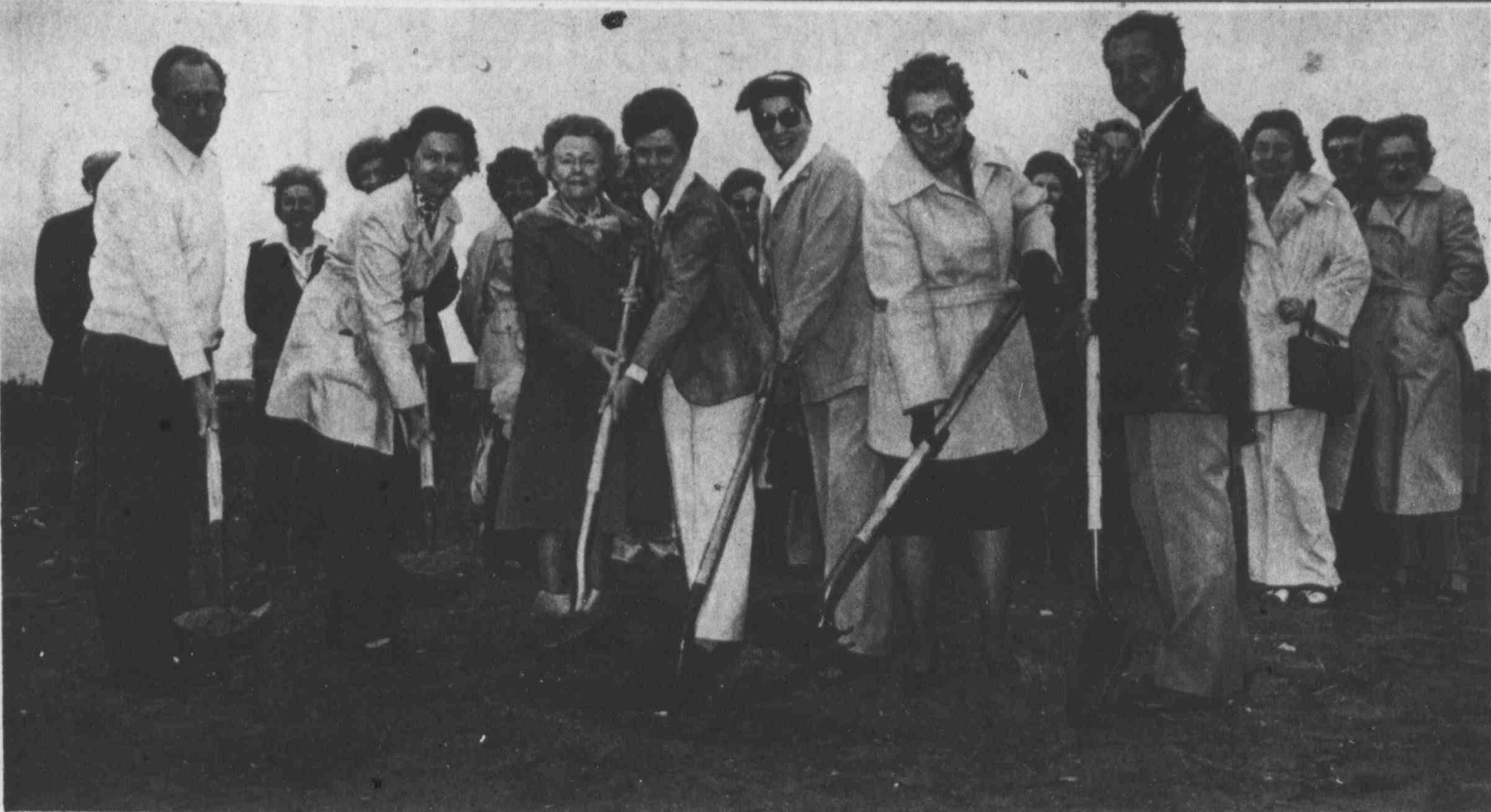
Members of the Permian Basin Duplicate Bridge Club break ground for a new bridge center to be constructed just south of Wadley Street near the City of Midland Swim Team's building. From left are A. G.
