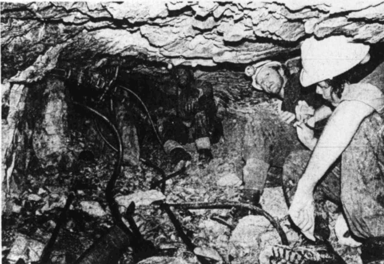
Jackhammer operators toil more than 2 miles underground, in tunnels often barely a yard high.
