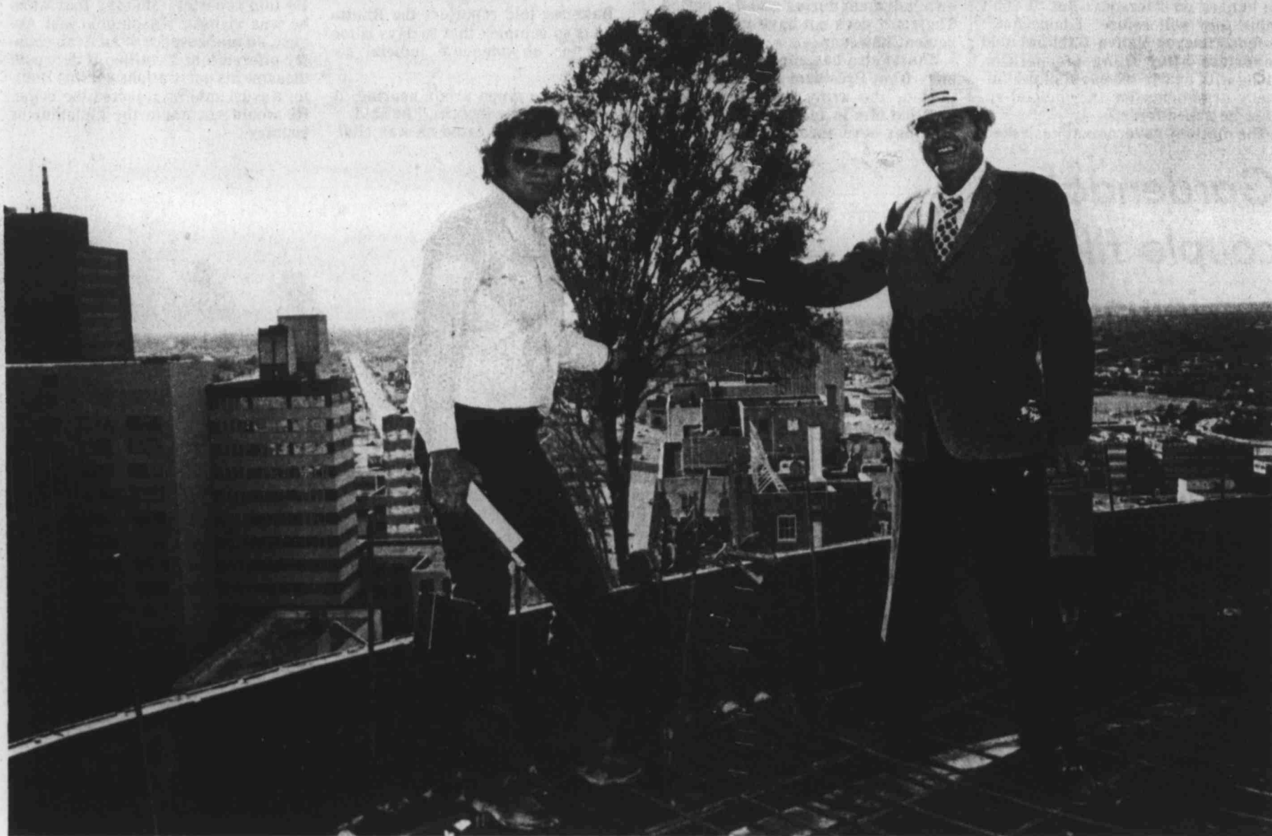
More than two months behind schedule because of recent weather conditions, the concrete top of the new Gibraltar Savings Association finally got poured Monday. On hand for the topping-off ceremony are, from left, Jim Farlee, carpentry foreman, and John Friberg, project manager for Mark Lee & Associates Inc., owner of the building. (Staff Photo)
