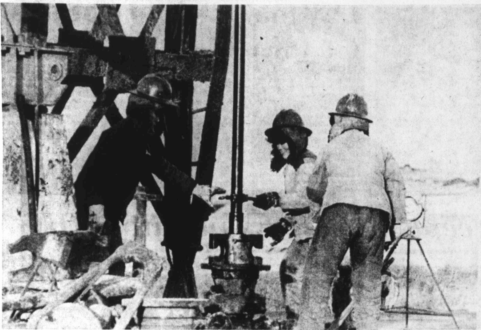
WOMEN WORKERS — Women workers in hard hats bring up oil tubes from an oil well where production has fallen off in the Sheng Li oil fields in the Shantung province of China recently. Engaged in "workover," or oil well repair and restoration, the all-woman unit does work many men would find arduous. (AP Laserphoto)
