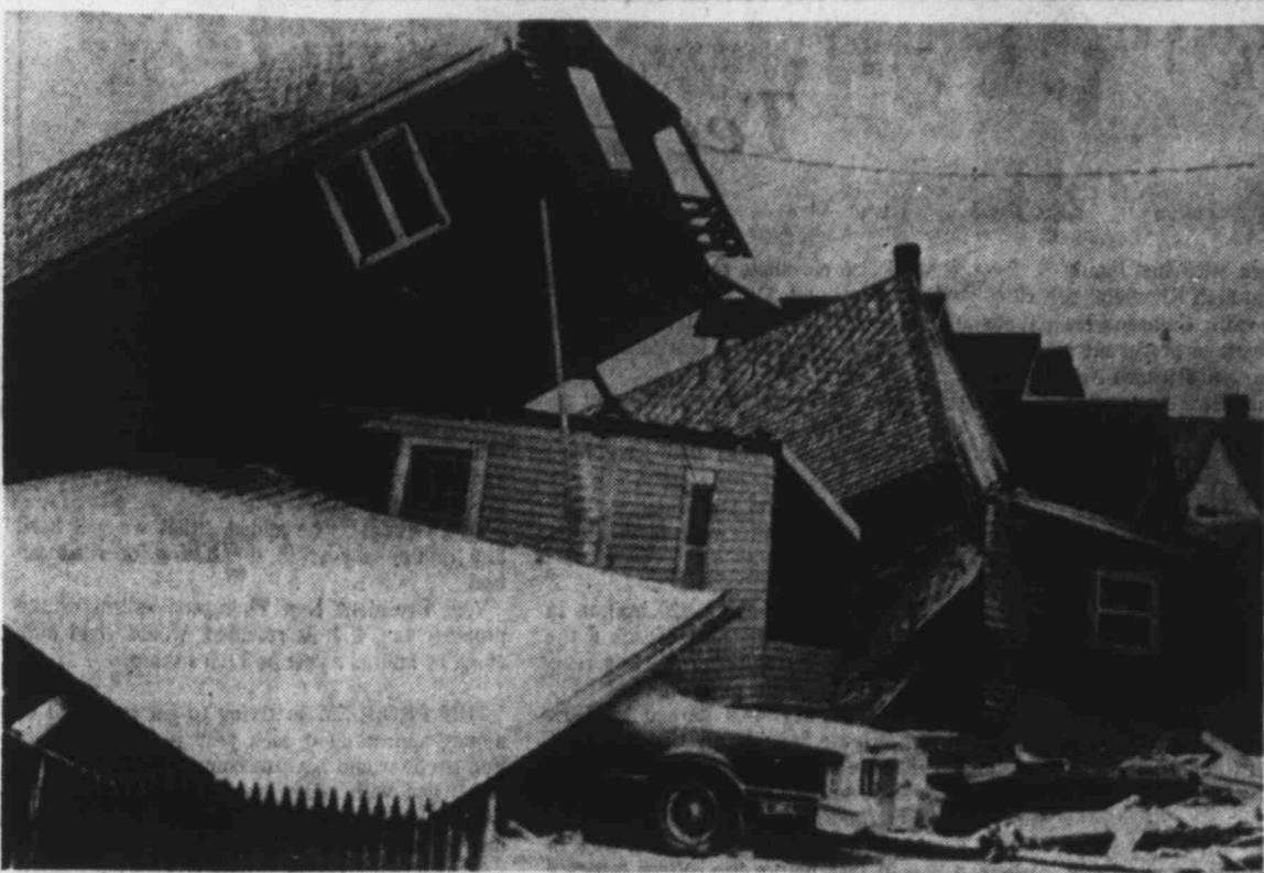
BLIZZARD DAMAGE — Ocean-front houses on Cedar Point in Scituate, Mass., lie scattered by snowstorms and high winds in this 1978 photo. Though an occasional bungalow still stands along Scituate's oceanfront, the most noticeable leftovers from the Blizzard of '78 are the numerous bills to pay for the damage. (AP Laserphoto)
