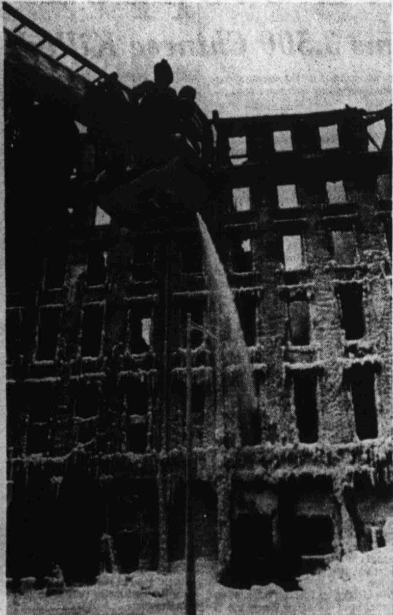
FACADE OF FROST — New York City firemen play stream of water on smoldering building already ice-covered in the Greenwich Village section of New York City Sunday. Fire fighters had been spraying the building since it first erupted in flame Wednesday night. Frigid temperatures coated the fire-blackened facade with white frost during the wet-down period. (AP Laserphoto)
